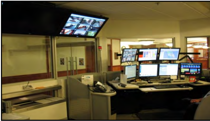
Radio room workstations, monitors, CCTV, radios
